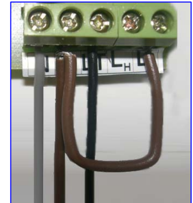
Wiring Photograph: Timer + Low Speed
