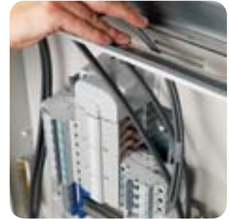
Unique trunking entry system
