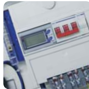
Metering fitted next to incomer within board
