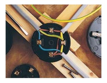
Providing the enclosure is fixed and accessible traditional junction boxes are acceptable
