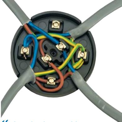
Junction boxes with screw terminals must be accessible for inspection...
