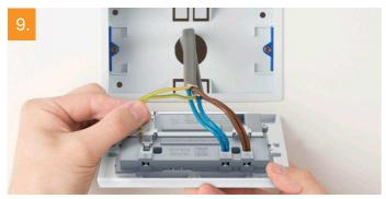
Place the blue wire(s) into the neutral terminal, brown into the live terminal and green/yellow into the earth terminal. The terminals on the socket are colour-coded to help locate the correct one.
