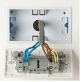
Alternatively, there could be two or three wires of each colour connected to each terminal.
