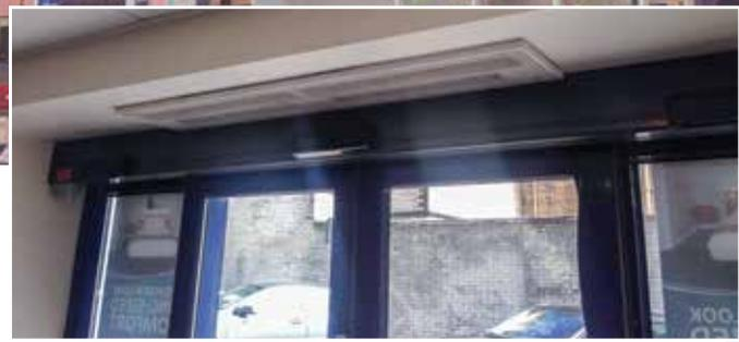
6kW heater used as an overdoor heater in a hotel
