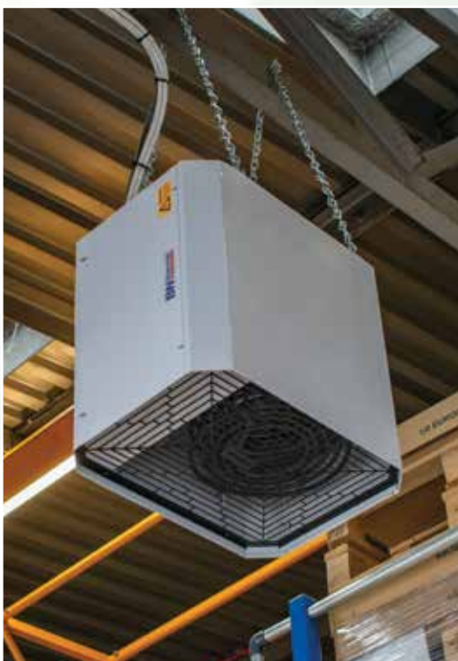
OUH2 Unit Heater suspended using hooks provided
