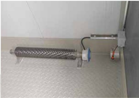
SWD mounted under SWG Guard An SWD guard is recommended when personnel have access to the heaters
