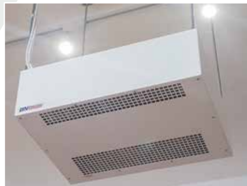
SMH heater suspended from drop rods
