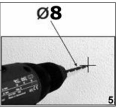
**5)** Using a drill bit with an 8 mm diameter, make holes in the wall on the positions that you marked in step 4.
