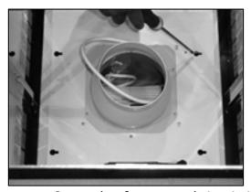
**14)** Lift the cooker hood fully over the framework, locating the framework into the screw holes shown in the picture.
