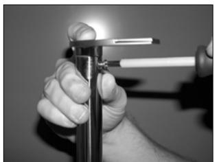
4) Place a bracket on either end of each handle and then using a screwdriver; fix the brackets with the screws provided. Make sure that these screws are fully tightened.
