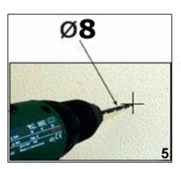
**5)** Using a drill bit with an 8 mm diameter, make holes in the wall on the positions that you have marked in step 4.
