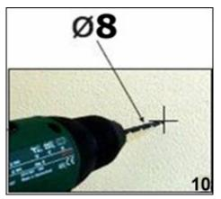
**10)** Remove the hood from the mounting bar and then using a drill bit with an 8 mm diameter, make holes in the wall on the positions that you have marked in step 9.
