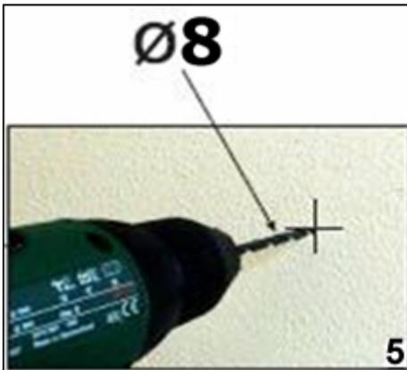
**5)** Using a drill bit with an 8 mm diameter, make holes in the wall on the positions that you have marked in step 4.
