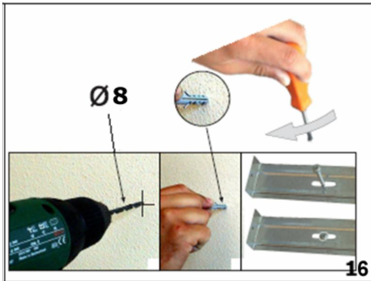
**16)** Using an 8 mm drill bit, drill out two holes on the pencil markings that you made in step 15. Insert screw anchors into the holes and then use a screwdriver to secure the fixing bracket to the wall.
