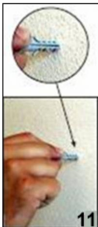
**11)** Insert screw anchors into the three holes that you have just drilled.
