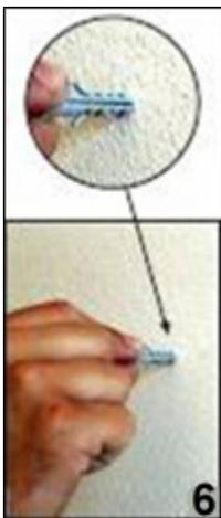
**6)** Insert screw anchors into the two holes that you have just drilled.
