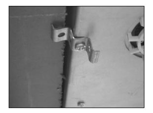
You should place the bracket on the underneath of the hob, in a position that is appropriate for the aperture that you have cut out. Using the screws provided, fix the bracket to the hob. These screws MUST be securely tightened.
