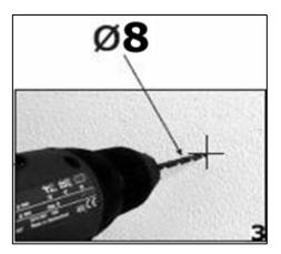
**3)** Using a drill bit with an 8 mm diameter, make holes in the wall on the positions that you have marked in step 2.
