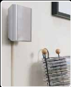
Use 16x8mm for speaker wires
