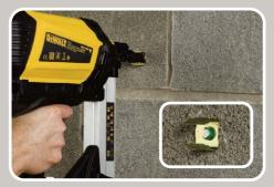
Shot-fired gas-nailing fixings are also popularly used for installing quantities of Safe-D® Clips.
