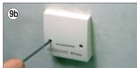
9b. Fit fascia plate using 2 x 30mm (M3.5) screws.
