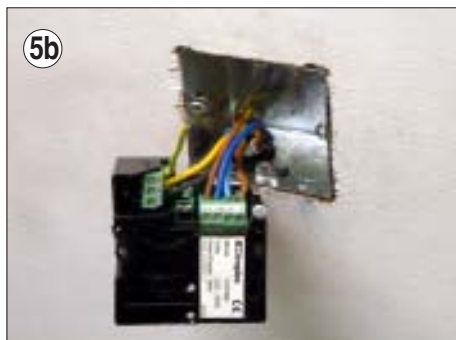
5b. Wire mains supply, appliance and pilot wire cables to pilot wire interface unit connectors.
