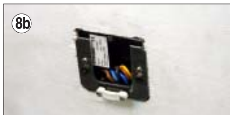
8b. Attach cable clamp bracket. Bracket is not required if the installer is fitting a fascia plate with holes centred.
