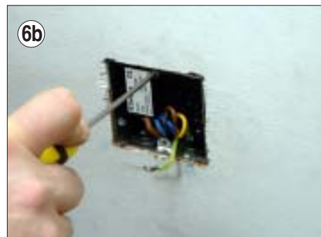
6b. Fit interface unit to back box and secure with 30mm screw (from fixing kit).
