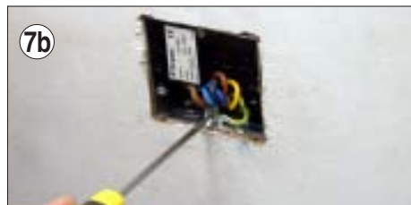
7b. Attach flying earth lead to lug on back box with 12mm screw (included in fixing kit).
