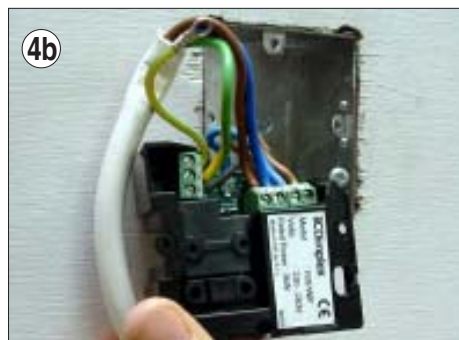
4b. Connect the cables to the interface unit and feed unit into back box. Guide the mains cable into place so that they don't exert excessive force onto the green connector blocks on the Interface Unit.
