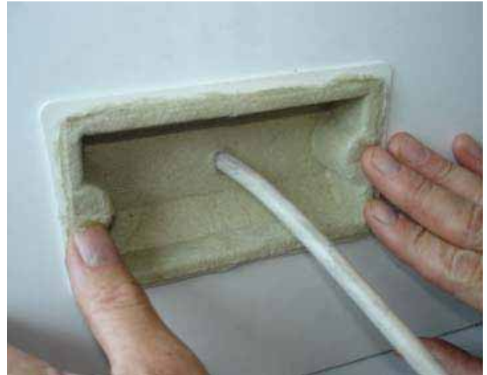
Firecap Switch/Socket Insert fitted into dry lining box
