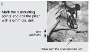
Fix the bottom then the top of the bracket.
