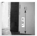
Mark the two wall bracket mounting holes with a 6mm dia. drill.
