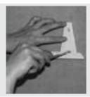
Mark the 2 fixing points of the wall bracket. Drill a 6 mm diameter hole and use the fixings supplied to fix the bracket to the wall.
