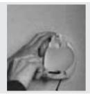
Mark the 2 fixing points of the base. Drill 6 mm diameter holes.
