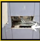
Pencil lines shown here are attempts from the dry-liner to cut around the back box on a party wall.
