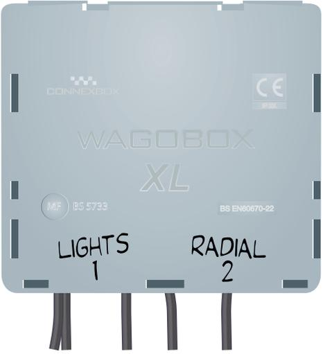
5. When two separate circuits are being supported no connections between the left and right side are permitted. Each side must be dedicated to one circuit only.
