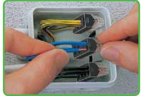
Removal: Hold conductor to be removed and twist alternately left and right while pulling the conductor.
