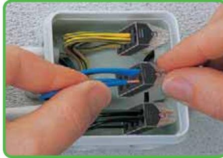
Connection: Insert stripped solid conductor fully!
