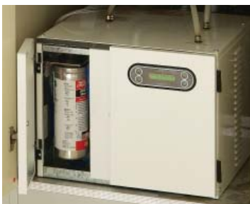
Hydrotap undersink assembly. The appliance must be placed in a horizontal position, as shown above.
