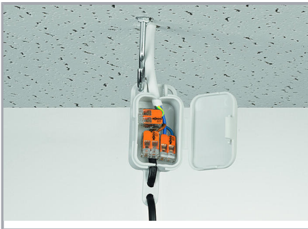
Pendant light connection in suspended ceilings
