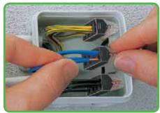
Connection: Insert stripped solid conductor fully!
