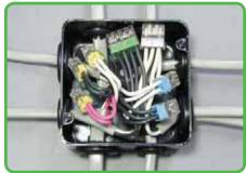
PUSH WIRE® connectors used in a junction box.
